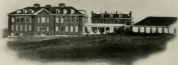
JORDAN HOSPITAL, PLYMOUTH, MASS. Harold Field Kellogg, Architect, Boston Carlisle & Connor, Elec. Contr's, Boston
